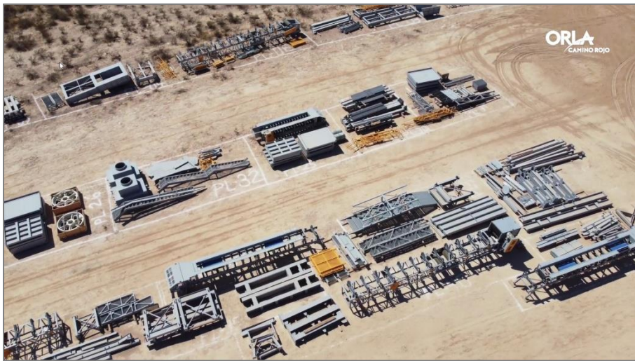
Figure 4: Process Plant Equipment Delivery and Laydown
