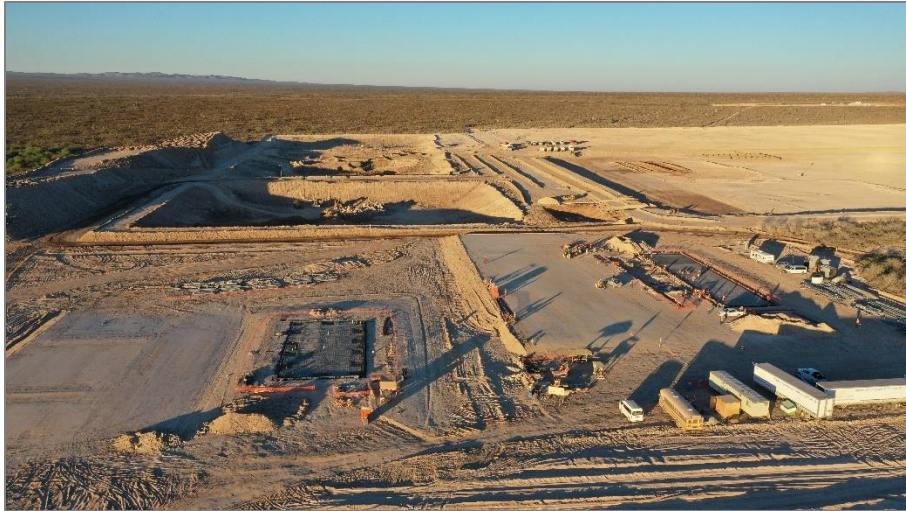
Figure 1: Excavation of Process Ponds and Preparation of Heap Leach Pad
