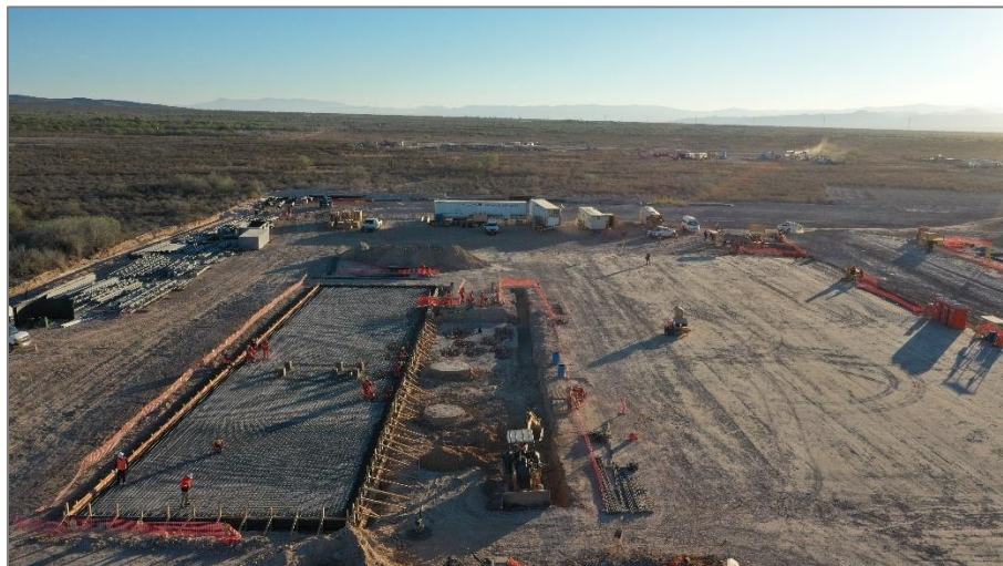
Figure 2: Preparation of Merrill Crowe Plant Area
