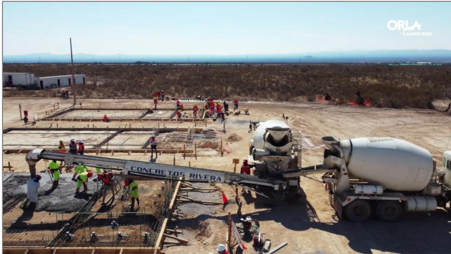
Figure 3: Preparation of Camp Area
